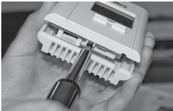
4. Align and secure the mounting base to the connection box using the two screws supplied.
